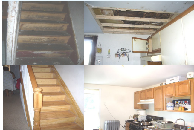
Before and after - the stairwell & kitchen at the Matthews'
