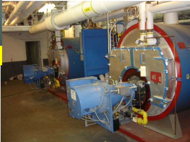
Logan Gardens boiler after repairs.
